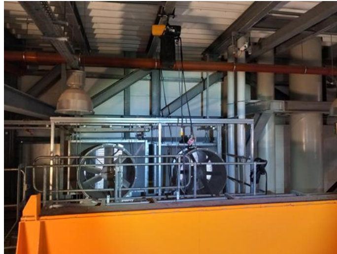
Figure 1-2 Turbine Hall Works
