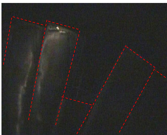
Figure 1: Boroscope photo of broken blade. Blades have been outlined with red dashed lines. Gap where part of the blade is missing can clearly be seen
