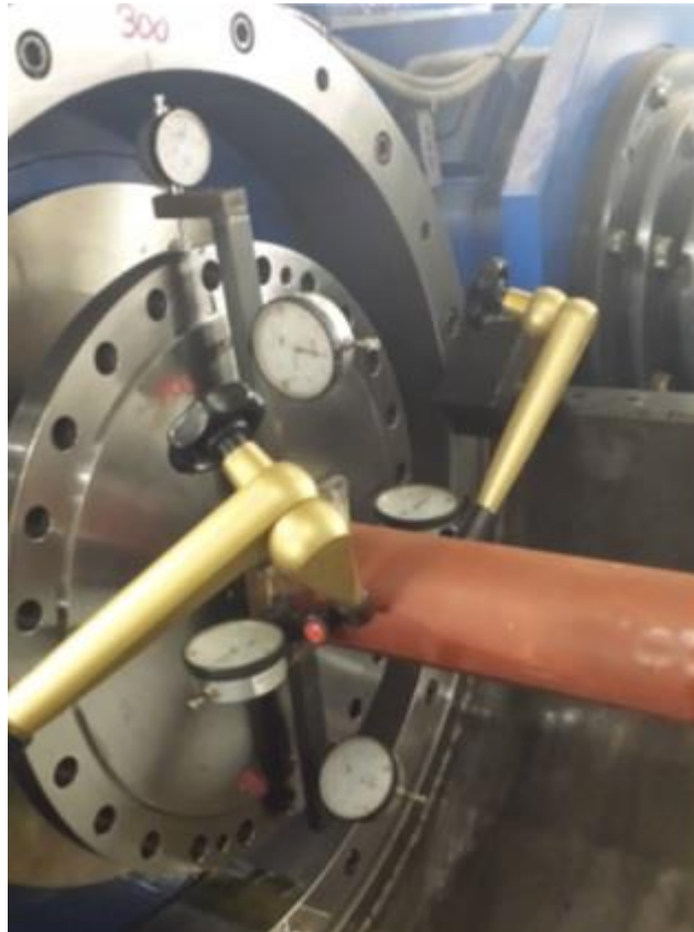
Figure 4: Movement monitoring devices attached to the TGM alignment bar confirming no movement of the turbine or gearbox when Flange X was opened.
