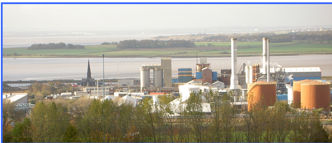
View from Weston Road
