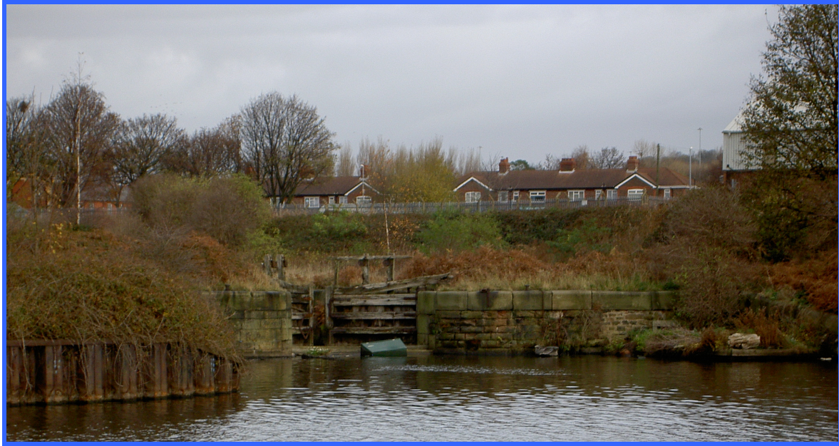
View of Millers Gate Lock from west bank of Weaver Navigation Canal
